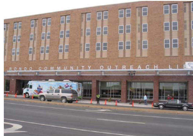
Library at street level, housing units on upper levels, one level parking sandwiched between Library and housing.
