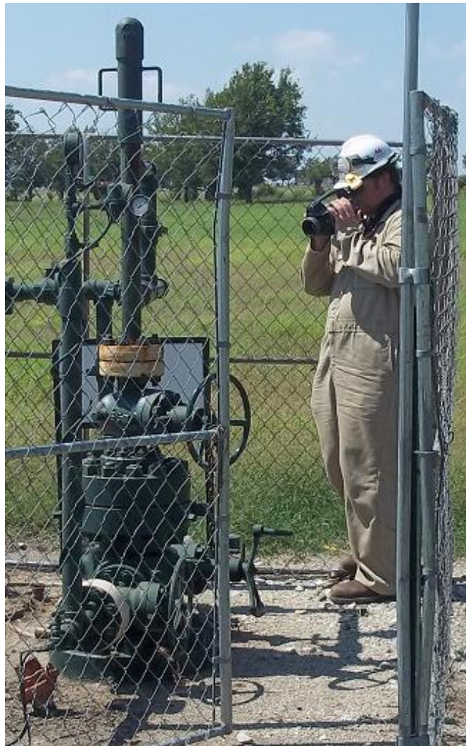
Field surveyor operating an IR camera at a well pad
