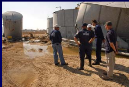
Damage from Hurricane Ike
