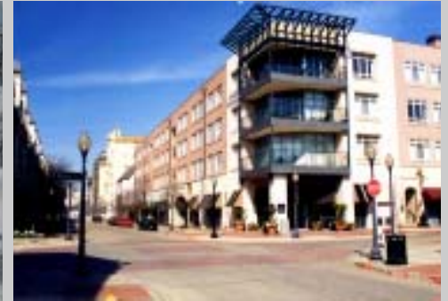
Façade projections and recesses may be dramatic or subtle. This façade combines both approaches.
