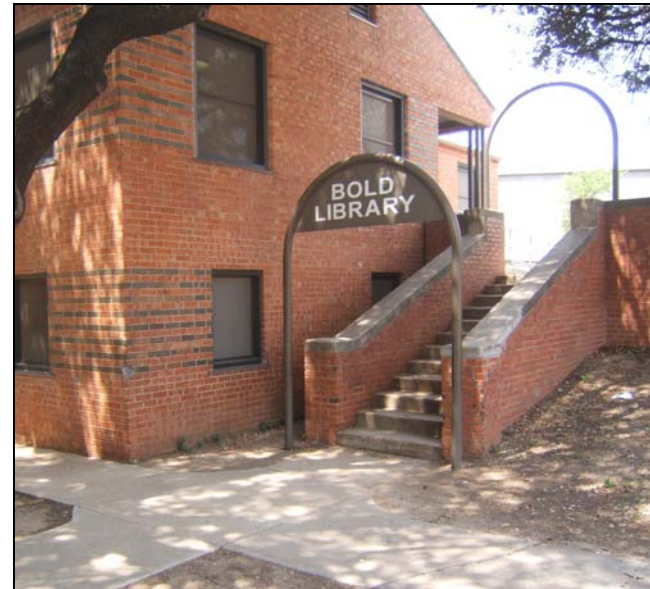
The Butler community has an on-site satellite library that opened in 1997 and is open five days a week. (Source: Fort Worth Housing Authority, 2007.)
