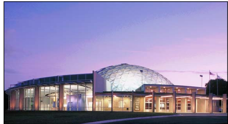
Originally built in 1958, Casa Mañana is a professional theater landmark in Fort Worth, providing live productions for adults and children. A $4.7 million renovation in 2003 transformed the structure into a 21st-century theater, creating a new 11,400 square foot steel-and-glass lobby to accommodate capacity crowds, and a stage and audience chamber featuring a modified thrust/proscenium stage configuration. The notable geodesic dome roof, designed by architect Buckminster Fuller, remains intact. (Source: Gideon Toal, 2003.)
