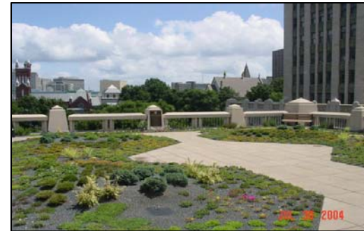
Green roof on Atlanta City Hall
