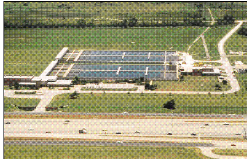
Aerial view of the Rolling Hills Water Treatment Plant and Central Laboratory. The plant was constructed in 1985 and the laboratory was constructed in 1998. Both facilities were funded by revenue from water sales and service charges. (Source: Water Department, 2006.)
