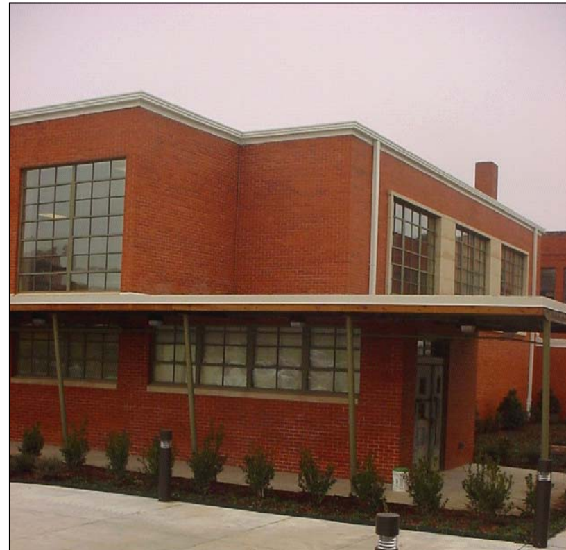
The Tech Fort Worth business and technology incubator, located at I-35W and Rosedale in the James E. Guinn School Complex, facilitates the growth and development of emerging technology companies in Fort Worth. This redevelopment project was funded in part by EDA funds. (Source: Tech Fort Worth, 2007.)
