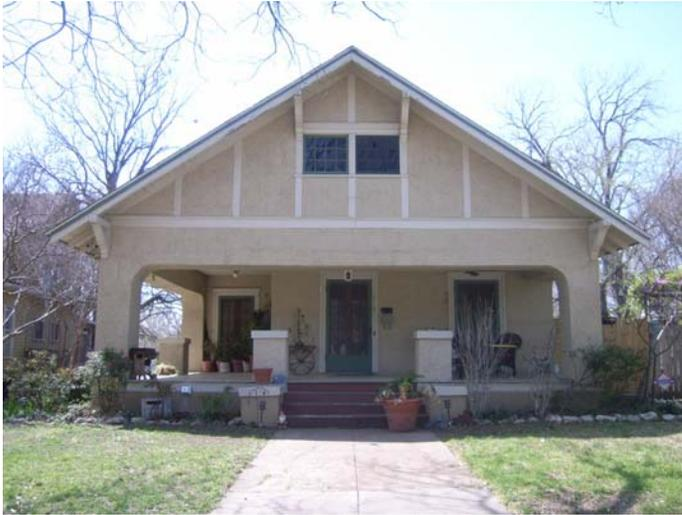
*LEFT: The half timbering in the front gable of this structure identifies it as an Arts and Crafts structure, but it also serves as expansion and ventilation joints for the stucco veneer.*
