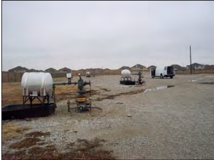
Figure 3.3-5. Site Documentation – Wells
