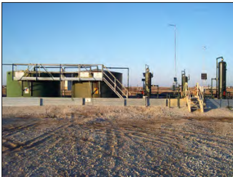
Figure 3.3-6. Site Documentation – Tanks and Separators
