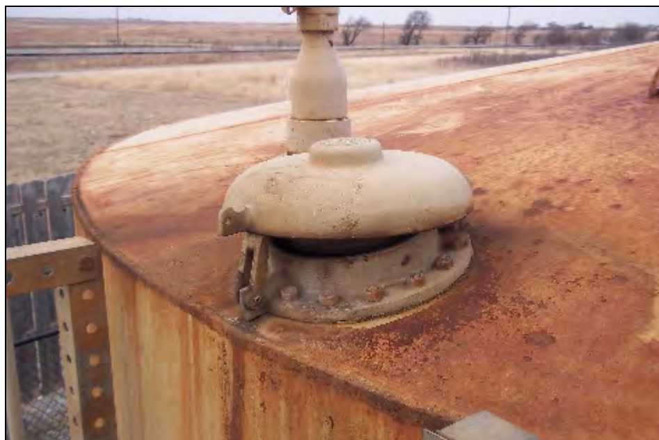
Figure 3.7-1. Thief Hatch Left Open
