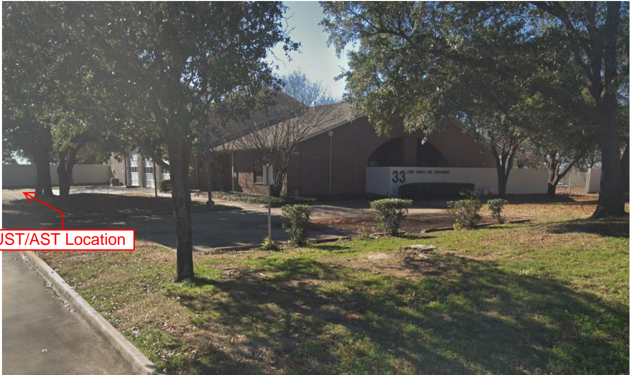
Fire Station # 33 – 14650 Statler Drive, Fort Worth, Texas 76155
