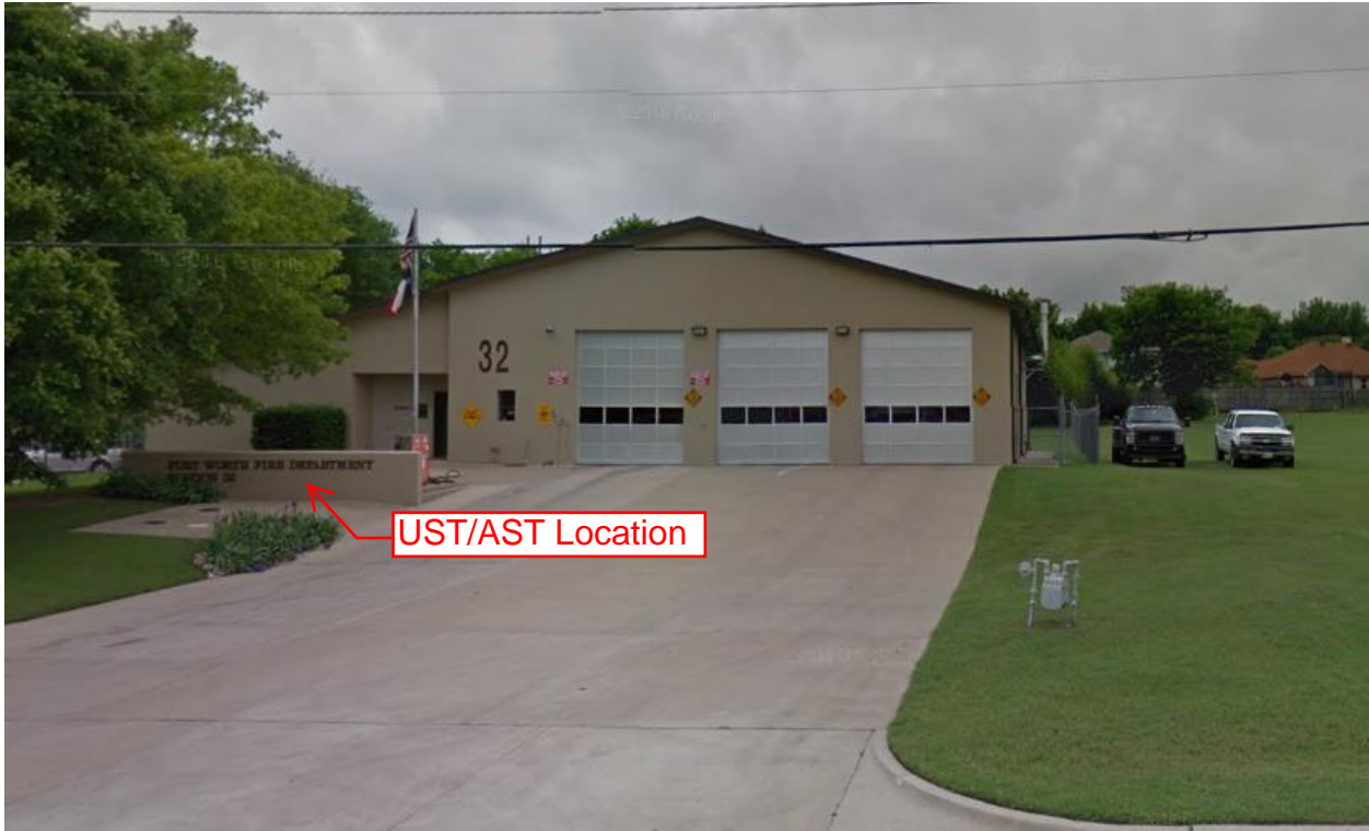
Fire Station # 32 – 10201 White Settlement Road, Fort Worth, Texas 76108
