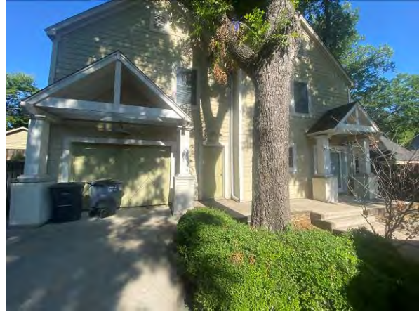
Exterior – rear elevation (main house at right, garage apartment at left)
