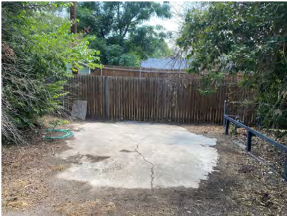
Exterior – uncovered parking area
