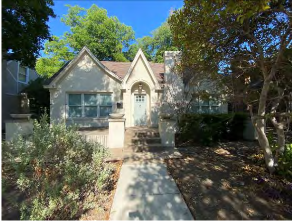
Exterior – front elevation (main house)
