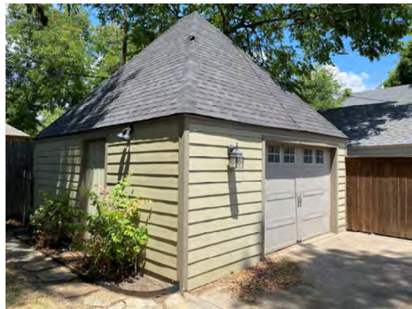
Exterior – detached garage
