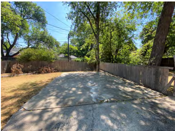
Exterior – uncovered parking area
