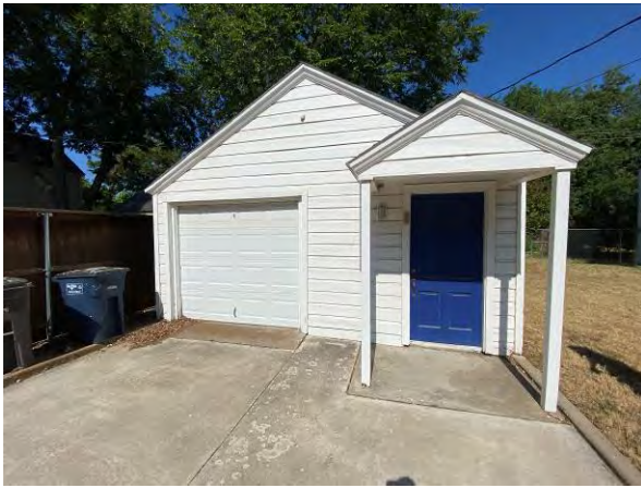
Exterior – detached garage/workshop
