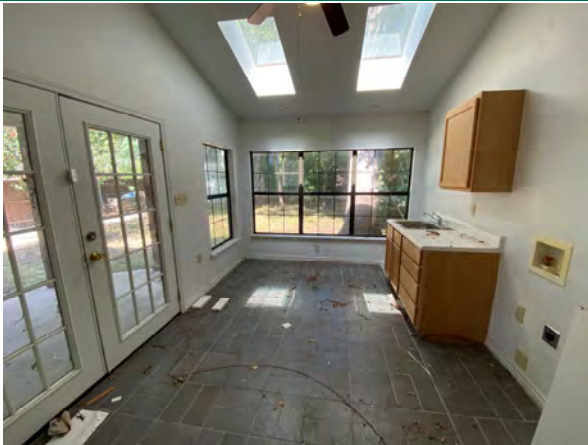
Interior – utility room
