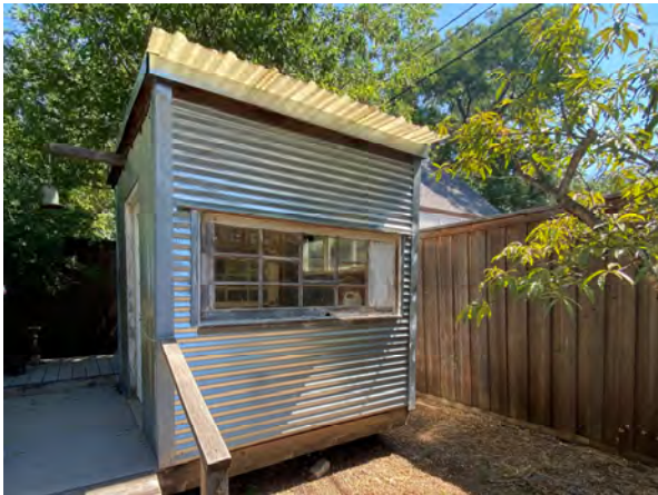
Exterior – unfinished shed
