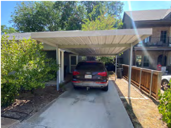
Exterior – attached carport
