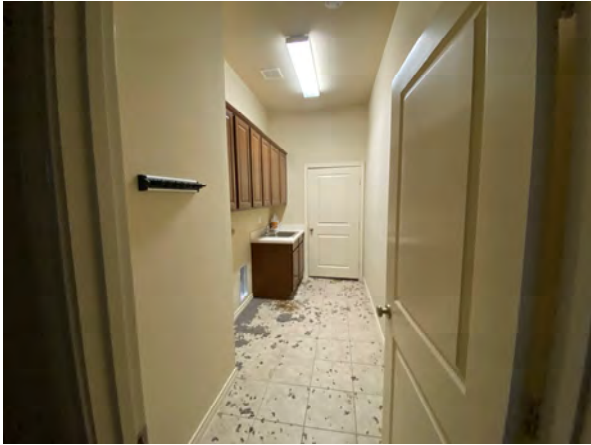
Interior – utility room
