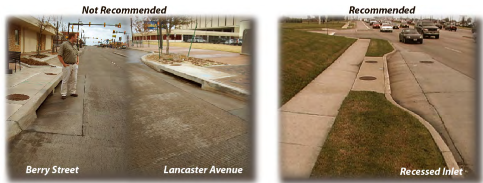
Exhibit 22: Drainage Inlet Design
