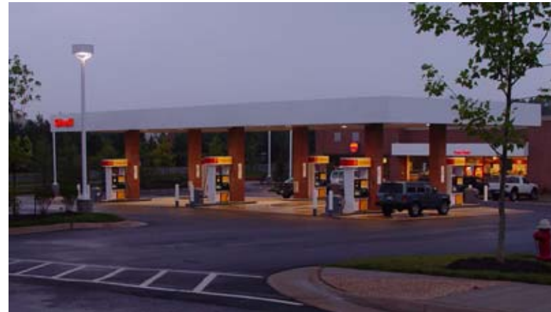
Example of service station down lighting
