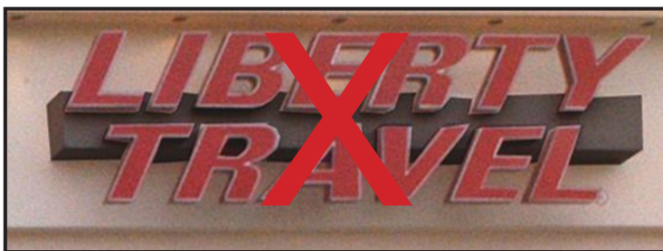
Above: Raceways less than 50% of the height of the letters and not painted to match the background are not allowed.
