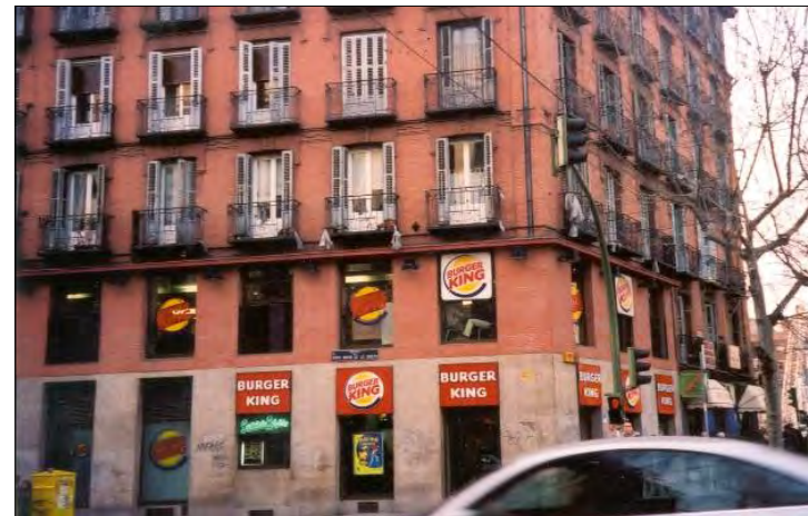
Repetitious signage on the same building frontage should be avoided.
