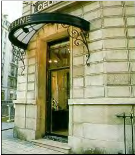
Signs can be incorporated into the design of both awnings and canopies.
