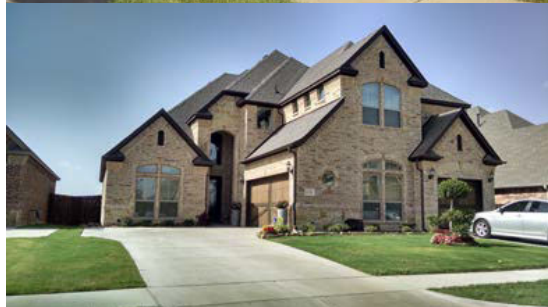
Images of a home with a J-Swing Garage from the front and side of home.
