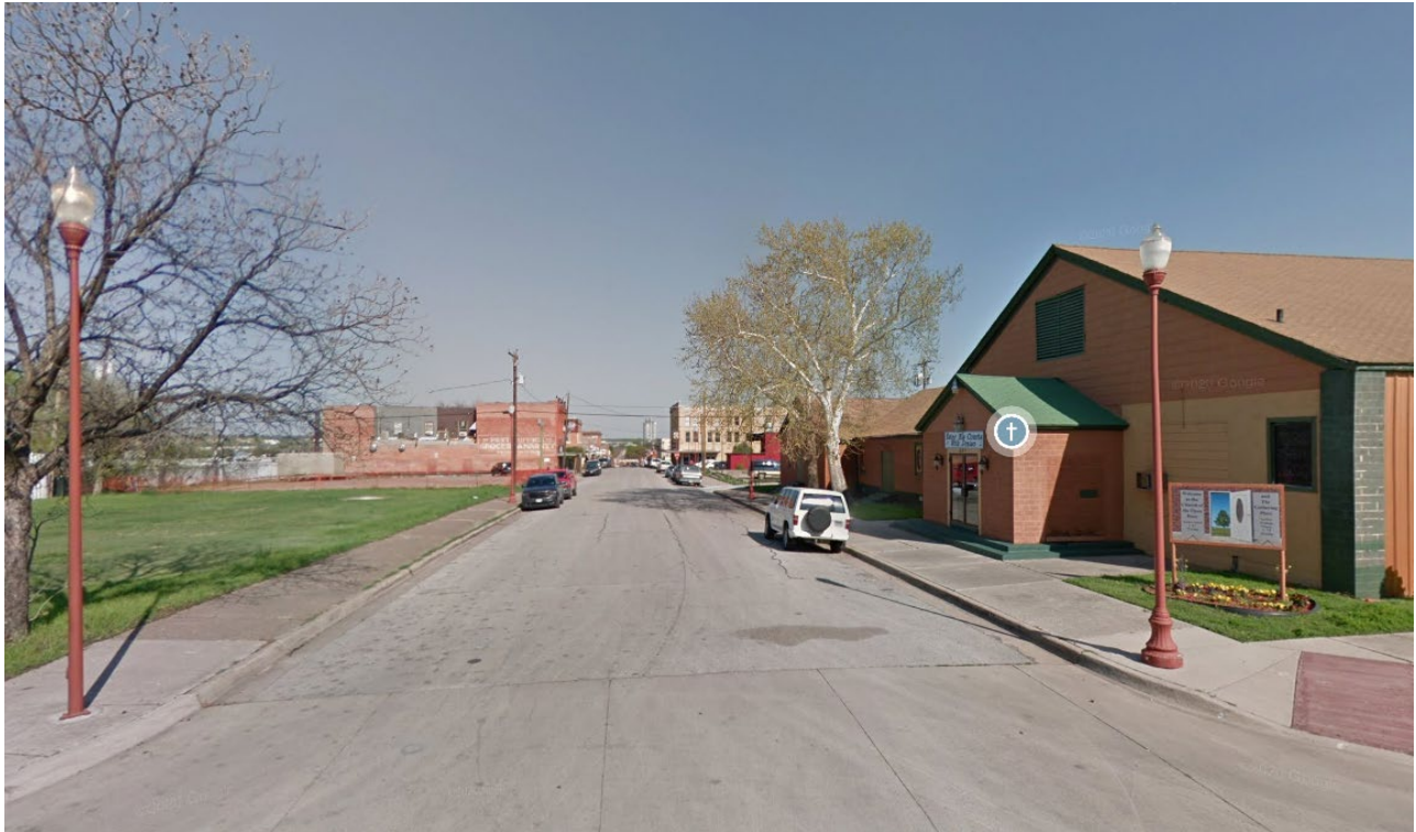
Fig. 13 – View looking east on W Exchange to the core.
