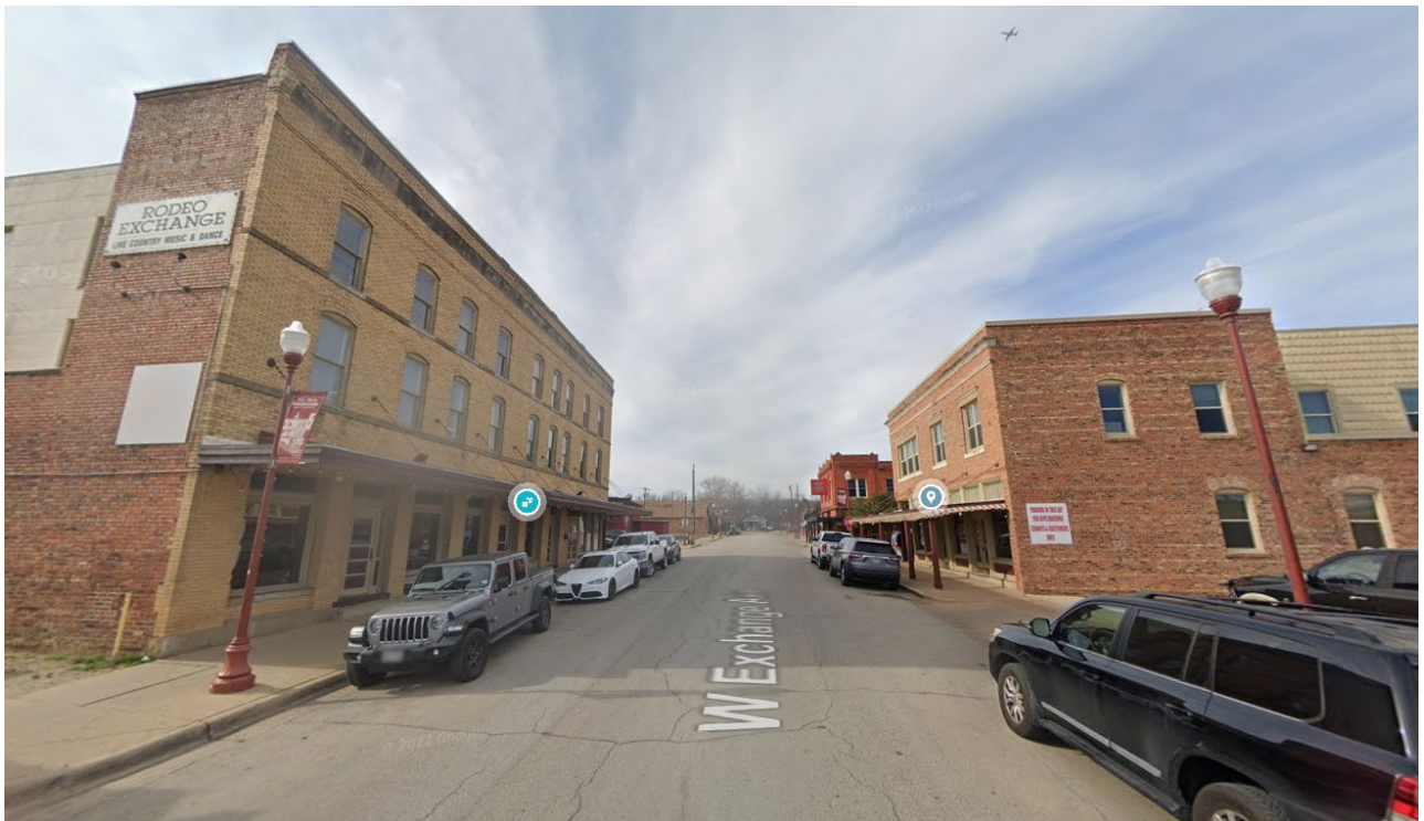
Fig. 12 – View looking west from Finney Ave.
