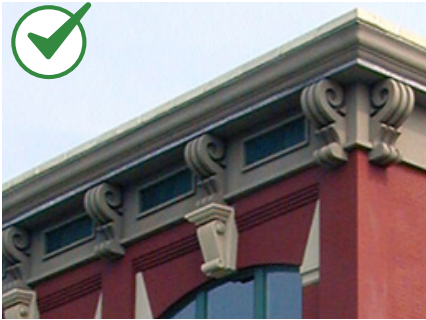
Restoration often involves individual building features such as this restored cornice.
