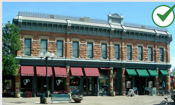
After: Original storefronts revealed.
