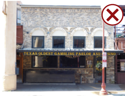
Many historic features, including the window openings and storefront, have been substantially altered on this property.
