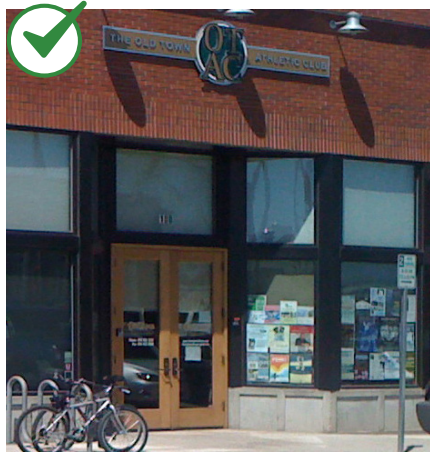
A simplified or contemporary interpretation of a traditional storefront may be considered where the historic storefront is missing and no evidence of it exists.
