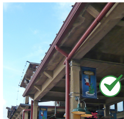
Preserve original materials.
