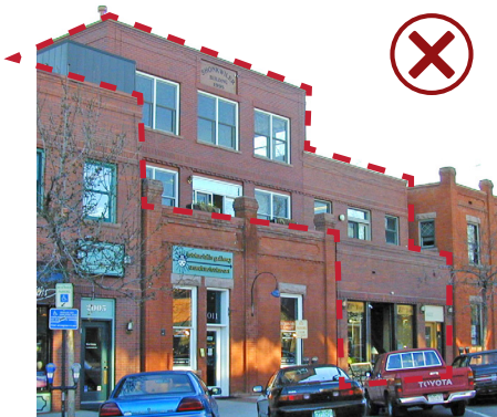
This three-story roof addition and side addition overwhelms the historic building due to its disproportion in mass and scale.
