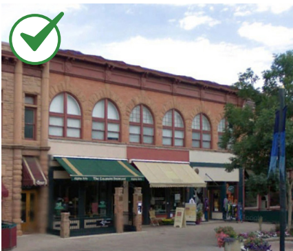
The removal of the inappropriate garage door and the rehabilitation of this commercial building successfully returns the property to the state that preserves the building's historic integrity.
