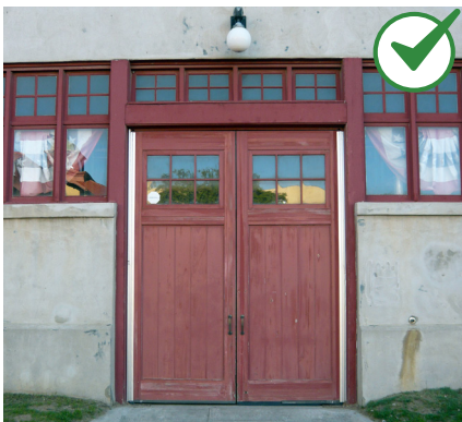
Preserve historic windows.
