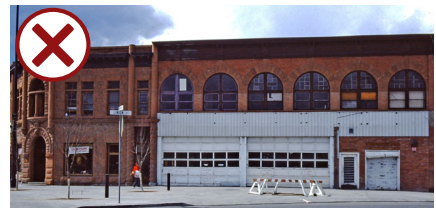
A change in use that requires alteration of key features, such as this, should be avoided.
