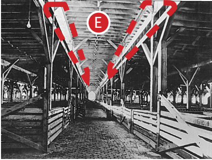
Early hog & sheep barns and pens were roofed with a “Y” frame construction with clerestories for sunlight and air flow (E).
