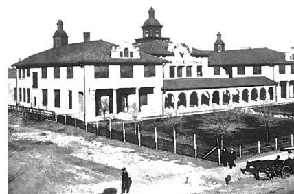
Southwest view of the Exchange building in the historic core of the Stockyards (ca. 1910).
