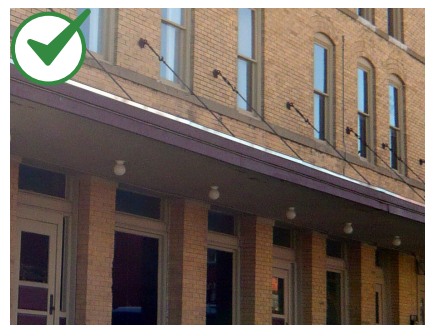
Appropriate canopy supporting mechanisms are wall mounted brackets, cable suspended columns or chains consistent with the style of the building.
