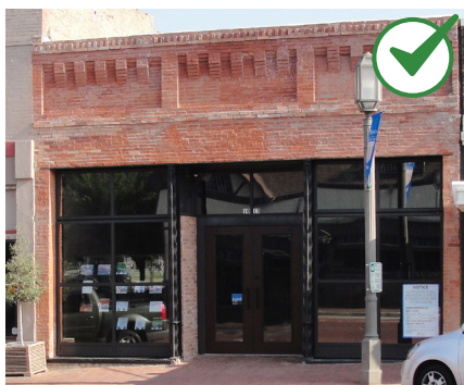
After: Historic storefront elements are exposed, following removal of non-historic stucco and other material.
