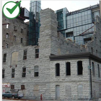
Some special opportunities may exist where a contemporary addition may be “inserted” into a shell of a historic structure.
