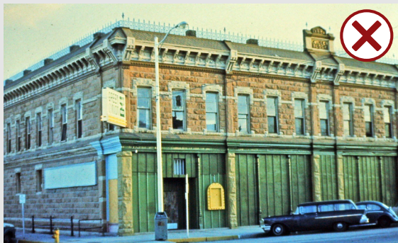
Before: Wood paneling obscures historic storefronts.
