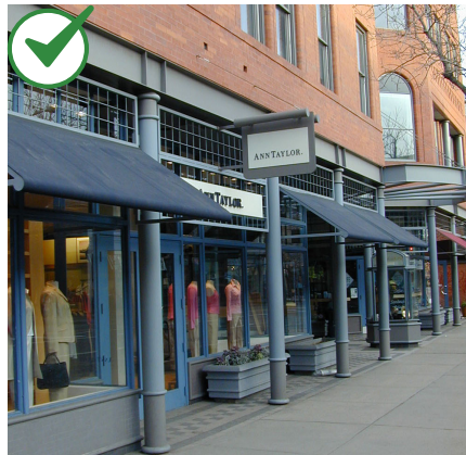
A compatible interpretation of a traditional storefront is appropriate where the original is missing.
