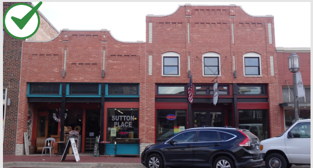
After: rehabilitation of historic building with reconstructed cornice, new windows and simplified interpretation of historic storefronts.
