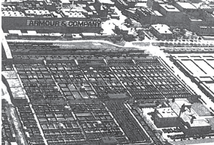
Buildings at the two meat packing plants step down in scale along the eastern edge (M).
