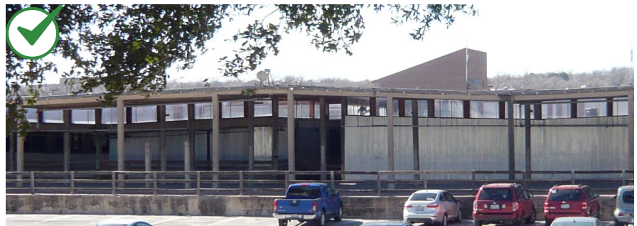
Maintain the original roof line and shape on a historic structure. The roof of the Stockyards Station building (the historic sheep and hog pen area) is a distinctive feature that should be preserved.
