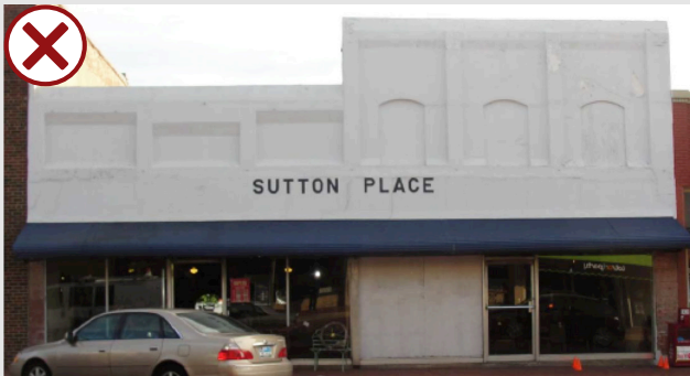
Before: moderately altered historic building
