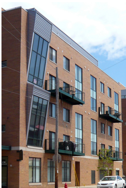
» Vertical expression (wall offsets and change in materials) » Horizontal expression (balconies and fenestration patterns)
