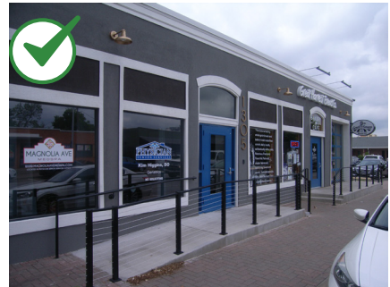
Preserve the integrity and character-defining features of a historic building when integrating accessibility solutions.
