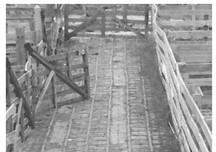
Raised brick thoroughfares provided footing for animals as they were moved.
