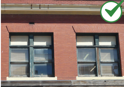
Repair, rather than replace, frames and sashes.
