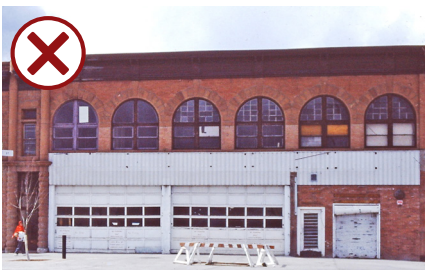
Remodeling the storefront of a historic building (Fort Collins, CO) to accommodate an auto repair shop is inappropriate. Storefronts were removed to make way for a garage. (Compare with the image below.)
