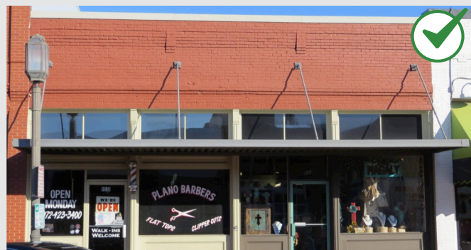
After: rehabilitation includes a reconstructed historic storefront, a historically accurate canopy and exposed original materials.
