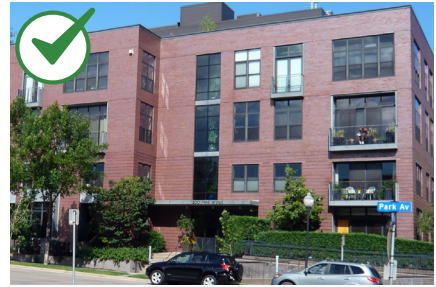
Use vertical and horizontal articulation design techniques to reduce the apparent scale of a larger building mass.
