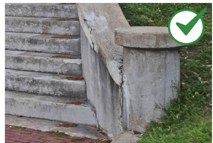
Maintain historic brick, stone and concrete masonry site walls.
