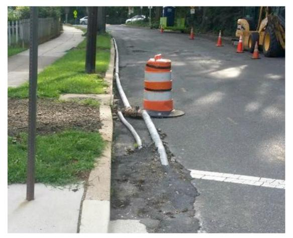
The temporary water line insures that you are not without water during construction. In the summer months the continuous flow keeps the water from becoming stagnant in the aboveground line.
