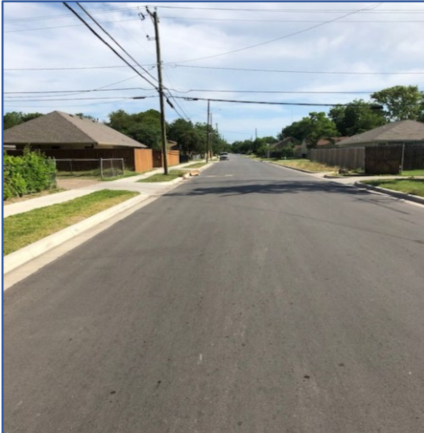
New Pavement and Concrete Curb & Gutter
