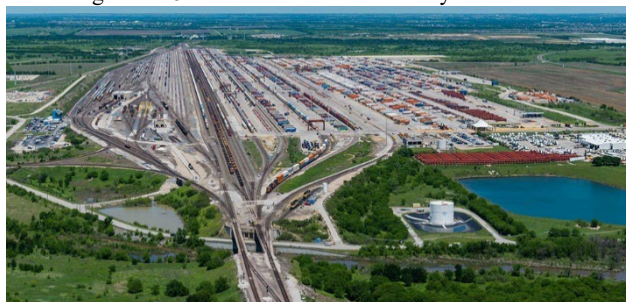
Figure IV-5: BNSF Intermodal Facility
