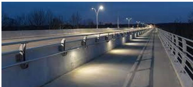
Figure IV-6: Pedestrian Lighting Example
