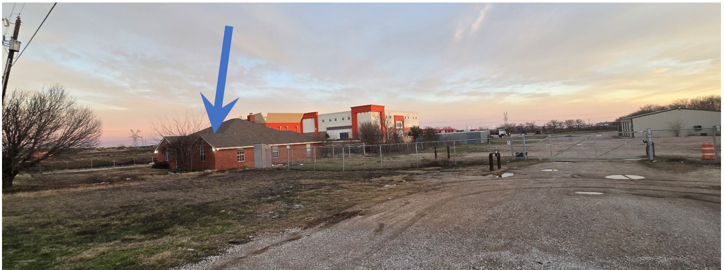
Figure 3: Site Photos taken by staff on 1/30/2025; view from 644 E Bonds Ranch Road
